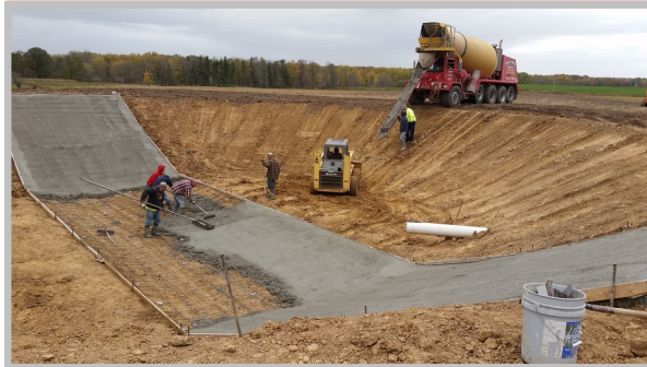
Concrete being poured into a constructed manure storage pit.
