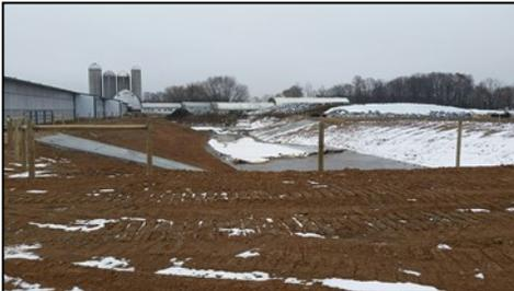
Above: Pankratz Farms, LLC expanded their existing clay-lined manure storage lagoon to allow 7-8 months worth of storage capacity. Concrete agitation pad ramps allow agitation equipment a place to operate without damaging the clay liner.
